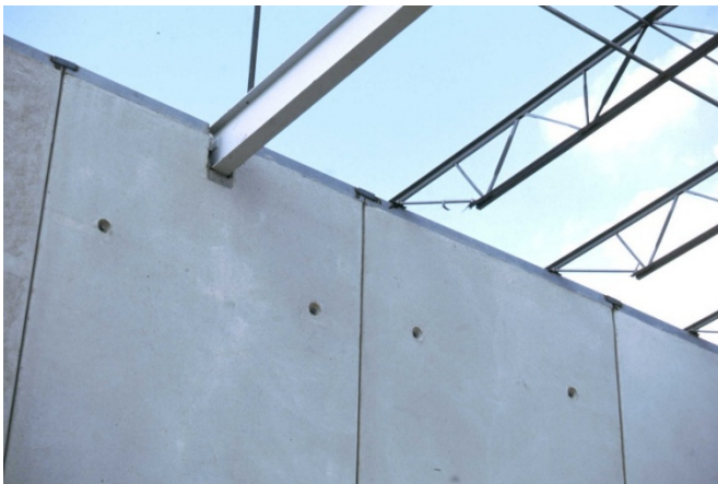
Figure 2: Loadbearing panels supporting a steel roof (Losch 2005)
